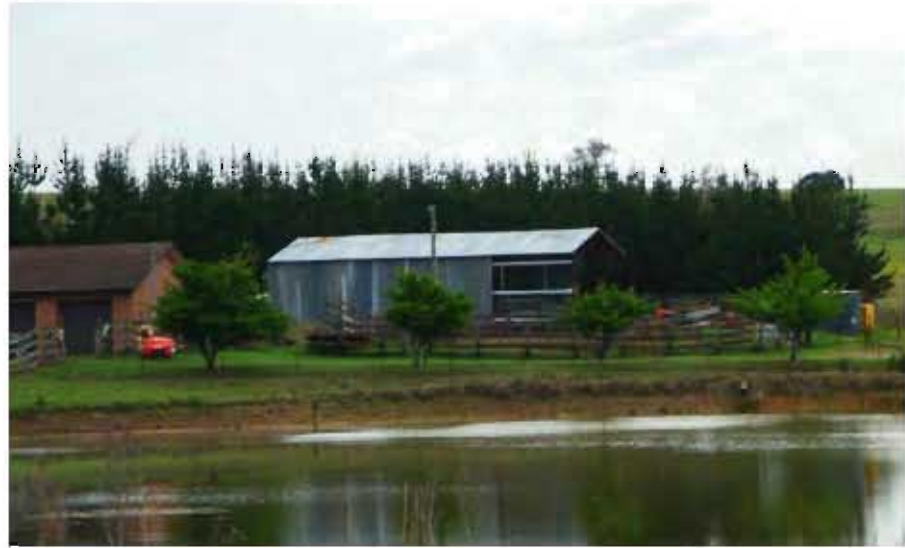
EXISTING METAL SHED TO BE DEMOLISHED
