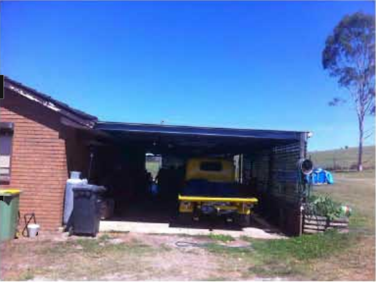
VIEW OF EXISTING RESIDENCE - REAR PERGOLA LOOKING WEST
